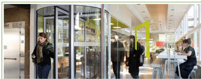
This revolving door in a Netherlands train station generates electricity to power a café's ceiling LED lights. The power is stored in super capacitors. The manufacturer, Royal Boon Edam Group, claims the door will provide 4600 kWh a year. There are many critics as well as fans of these human-powered doors.
